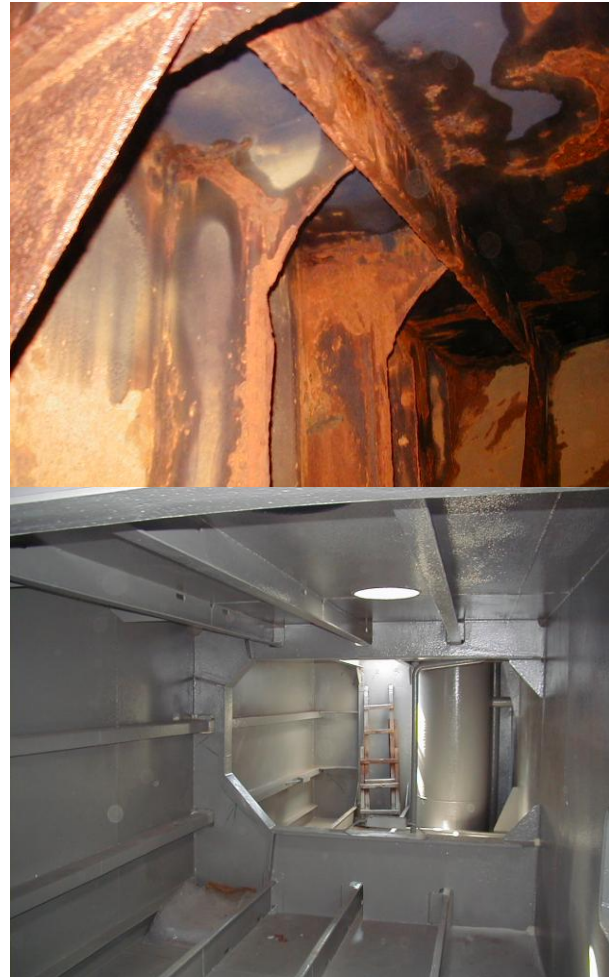
Coating rating only for Ballast Tanks
